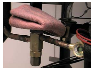
Figure 5-4 TXV Removal
